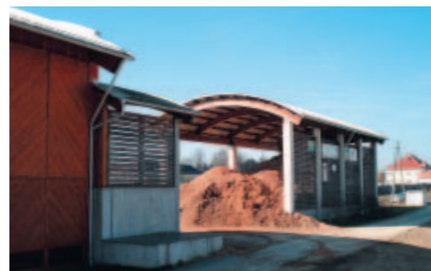
Figure 29: Building for wood chip storing. Source: BE 2020+, 2010.
