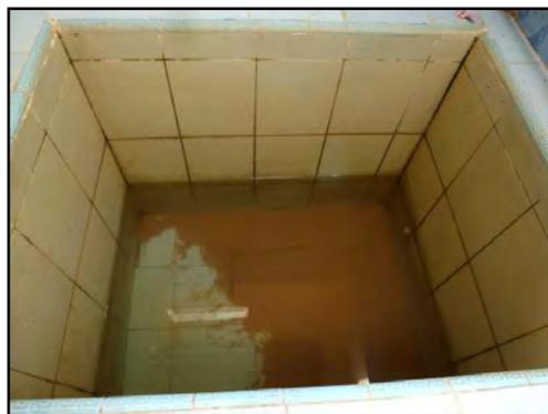
**Fig. 42: Sediments in a water tank in the bathroom of our guest house (own picture)**
